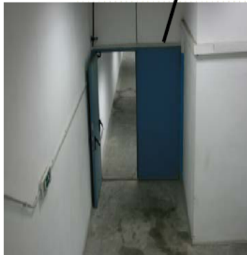
Direct emergency exit to the surface
